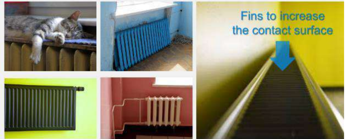
A water to air heat exchanger
