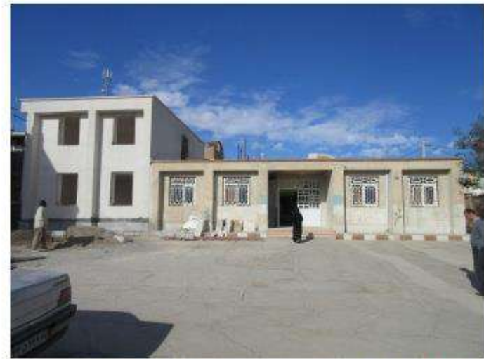
b) The retrofitted single-story unconfined URM building adjacent to the appendant newly-constructed confined URM building; both of which experienced very fine cracks
