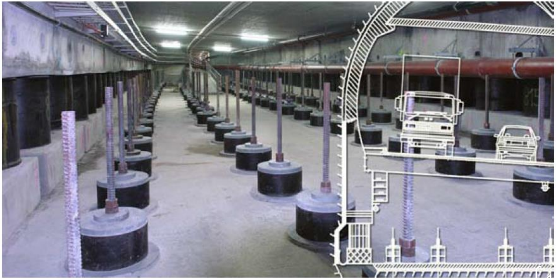
Fig. 20: Chienberg Road Tunnel after completion: “Modular Yielding Support”
