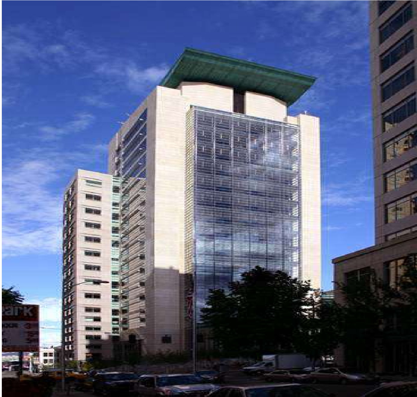
U.S. Federal Courthouse, Seattle •
