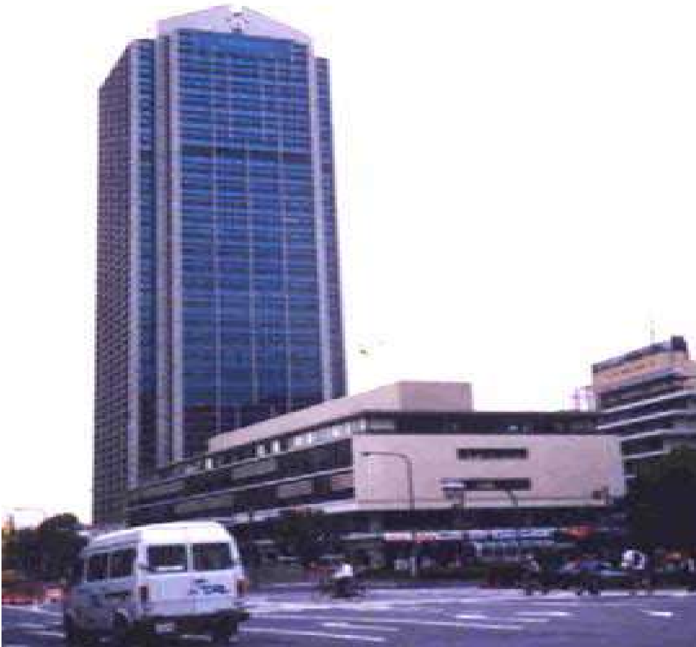
Kobe Office Building, Kobe •
