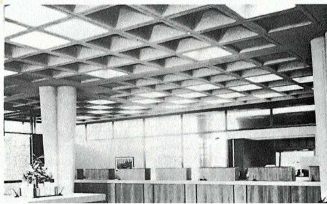
Waffle plate two-way structural system
