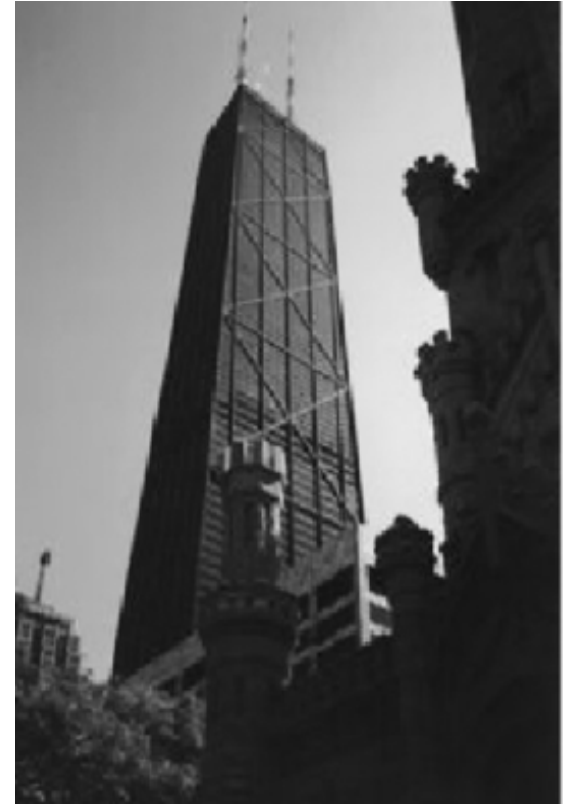
John Hancock Center, Chicago, USA
